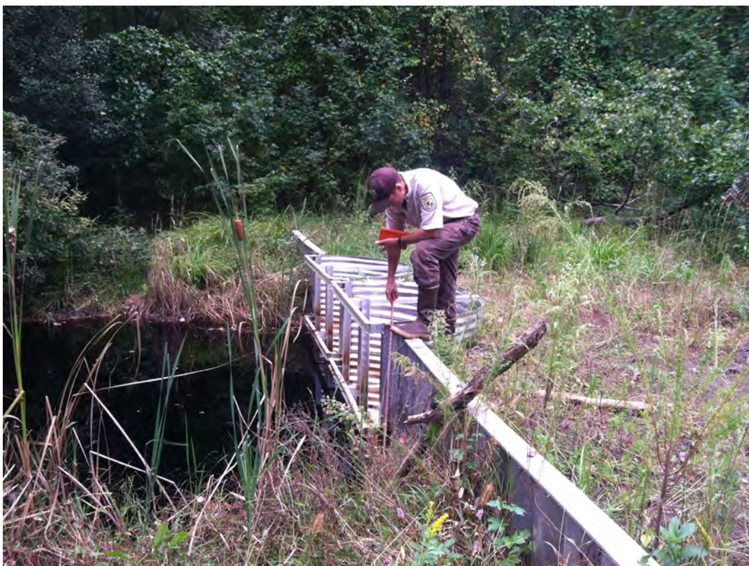
Figure 20.1 Water control structure to block a drainage outlet in Great Dismal Swamp, VA
