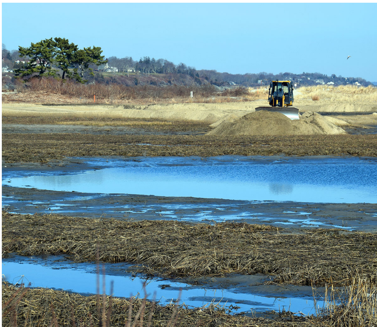
Figure 3.1 Adding sediment to Maidford Marsh at Sachuest Point National Wildlife Refuge in Rhode Island
