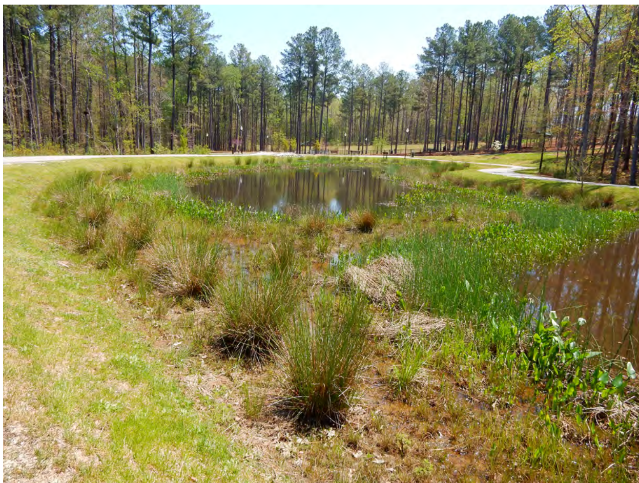
Figure 15.1 A stormwater treatment wetland in Apex, NC
