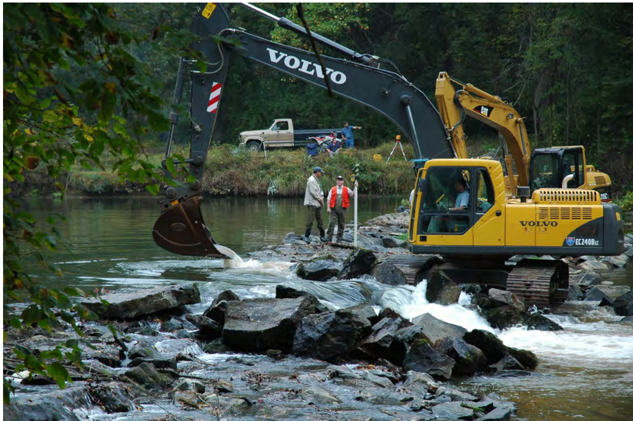
Figure 24.1 Dam removal on Octoraro Creek, MD
