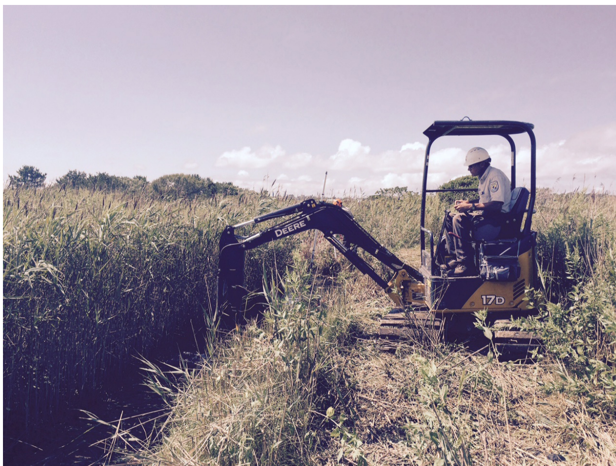
Figure 1.1 Digging ditches to improve drainage and remove invasive plants in Sachuest Point National Wildlife Refuge
