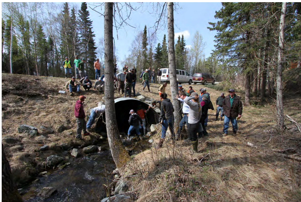
Figure 24.2 Fish-friendly culvert in Anchorage, AK
