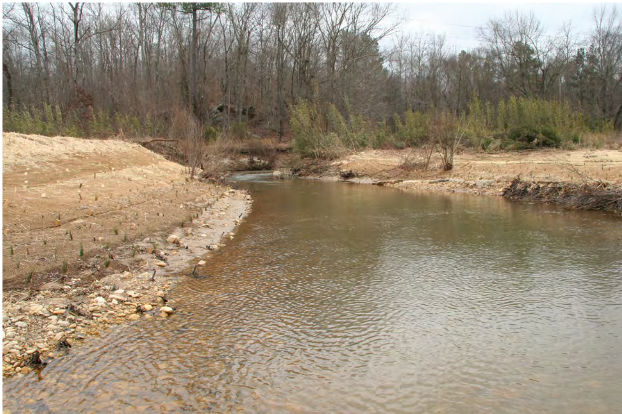
Figure 25.1 A regraded and planted stream bank at Raccoon Creek, GA
